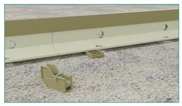
Insert the pin into the Clamp body, ensuring the tie is loose enough to allow the body to slide along the pin.
